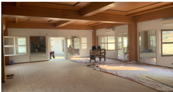
Thi công trần, lát sàn nhà hàng Việt Nam dự án Movenpick Resort Cam Ranh Construction of ceiling and floor of Vietnamese restaurant of Movenpick Resort Cam Ranh project
