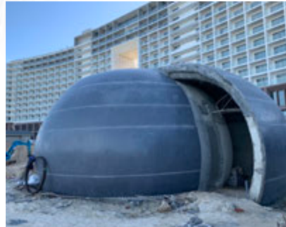
Thi công dự án Movenpick Resort Cam Ranh Construction of Movenpick Resort Cam Ranh project
