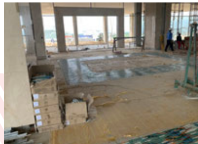
Thi công ốp lát nhà hàng Việt Nam dự án Movenpick Resort Cam Ranh Construction of Vietnamese restaurant tiles Movenpick Resort Cam Ranh project
