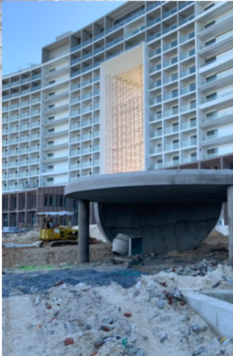
Thi công dự án Movenpick Resort Cam Ranh Construction of Movenpick Resort Cam Ranh project
