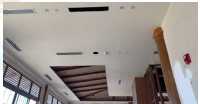
Thi công trần nhà hàng Việt Nam dự án Movenpick Resort Cam Ranh Ceiling construction of Vietnamese restaurant Movenpick Resort Cam Ranh project
