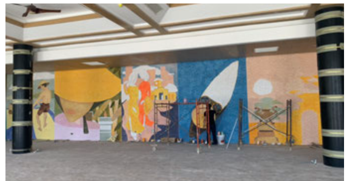
Thi công ốp lát tường nhà hàng Việt Nam dự án Movenpick Resort Cam Ranh Construction of wall tiles for Vietnamese restaurant Movenpick Resort Cam Ranh project
