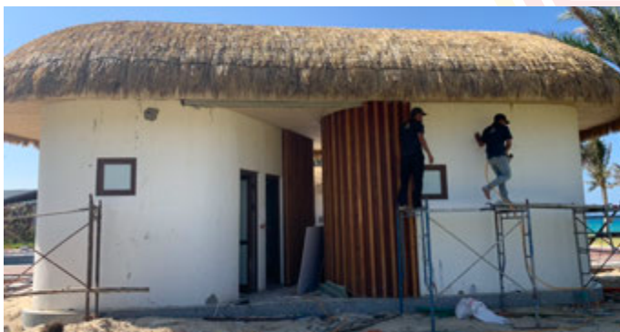
Thi công dự án Movenpick Resort Cam Ranh Construction of Movenpick Resort Cam Ranh project
